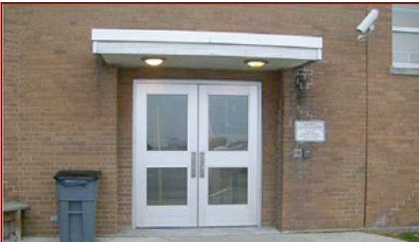
Existing Vestibule Entrance
