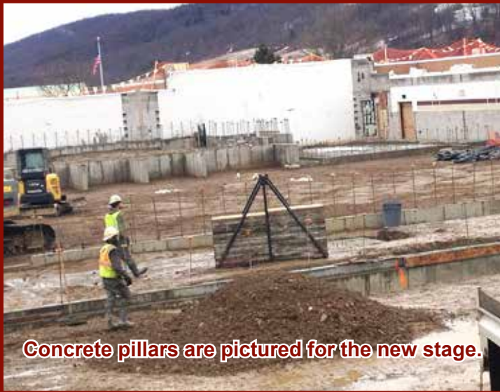
Crews back fill foundations for new locker rooms.
