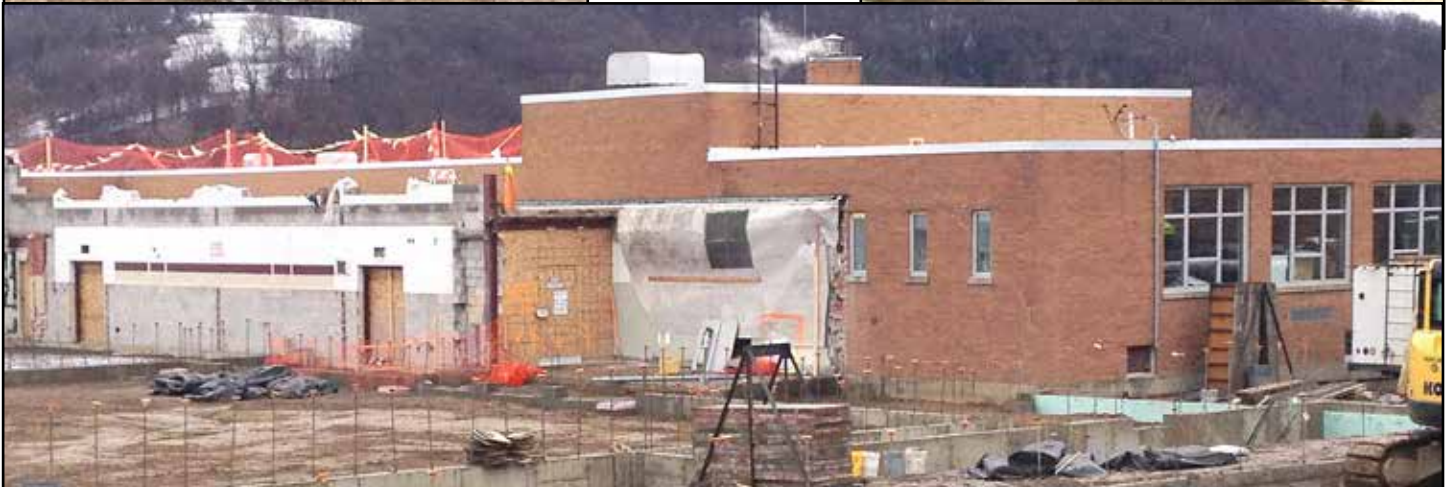
BELOW: The covered area is the old corridor to gym and cafeteria. Wall to the left is the inside wall of the "old gym."
